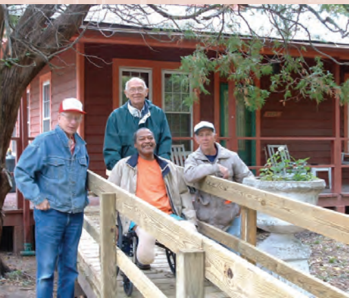
From left to right, Dean Hanshew, John Morris, and Russ Luecke of Bellefontaine UMC in the Missouri East Conference test out the new ramp with Keith Graffin, who will have a much easier time getting into his front door. The Bellefontaine Church was challenged in the Academy to be more inclusive, both in the church and in the community.
